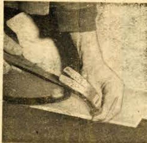
Firm pressure on the board with foot or knee, and also on nail will give you the best results.
