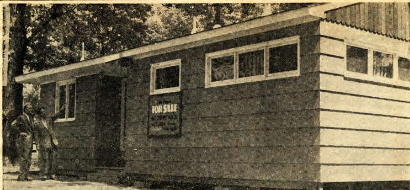
Salt Lake area Vocational School officials, Jay Nelson, left, and Algot E. Anderson, inspect four-room house constructed at 4th South and 6th East by students as a training project. House has kitchen, dining room, and two bedrooms.
